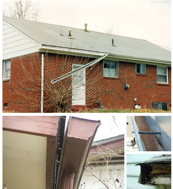
Above: Traditional attachment systems such as this gutter attached with spike and ferrule often fail during the harsh winter months because the fascia board is rotten and can no longer support the weight of ice and snow. Top Right: “Proud” spikes indicate that the fascia board may be compromised and no longer solid wood. Bottom Right: Over time this trapped moisture from spikes causes wood rot to the fascia and rafters.
